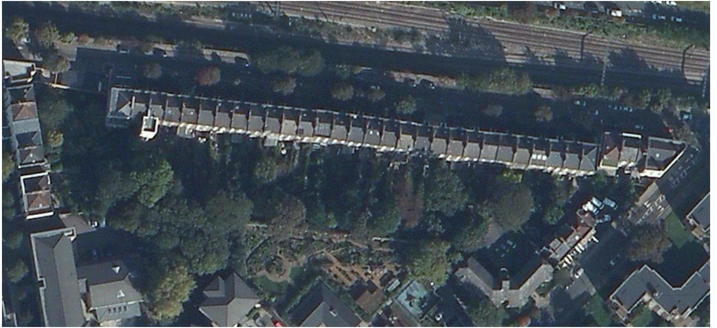
Image 1 - Aerial view of the site and surroundings
